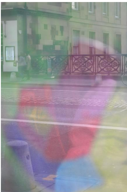
Details from 2017 windows, with George IV Bridge reflected in glass
